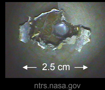
Shuttle radiator damage, 2007
